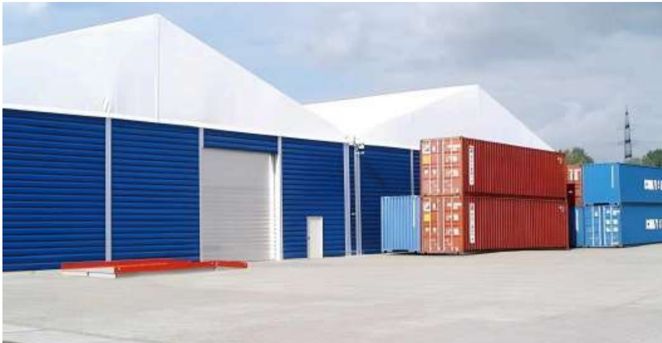
● Container Cargo Storage Tent
