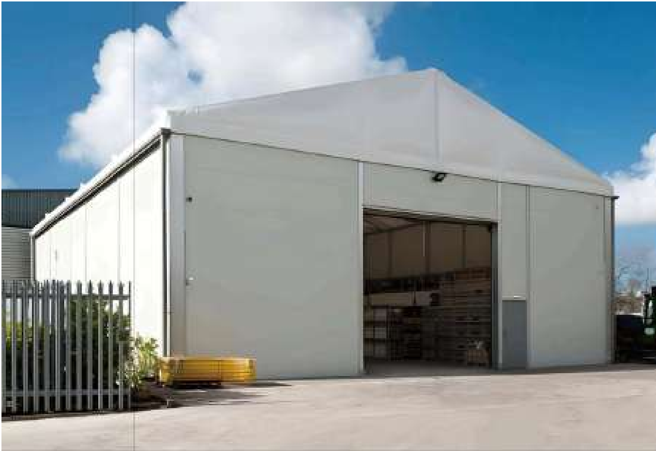
● Zhaotong City, Yunnan Province Building Materials Factory Storage Tent
